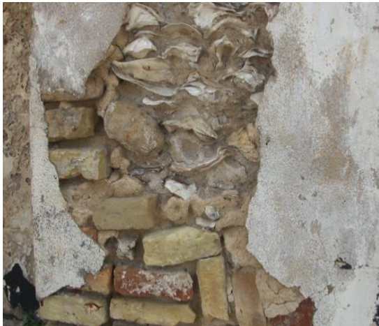
Figure 4.2 Fort Keta's Wall An exposed wall, washed away by the sea, shows the use of foreign brick and local oyster shells in the building's walls.
